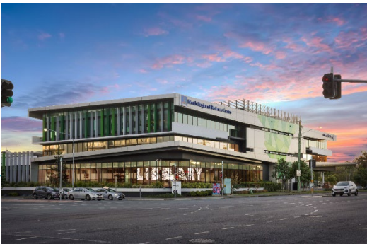
NORTH REGIONAL BUSINESS CENTRE Brisbane City Council Library and Councillor offices
