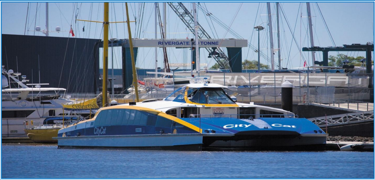
Rivergate – New CityCat Maintenance Facility
